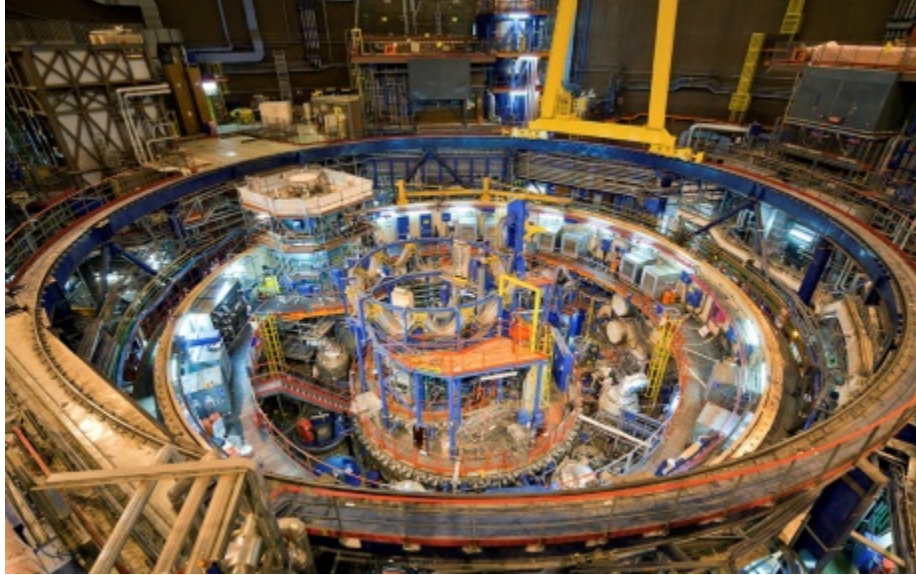
Figure 57 Superphénix during construction
